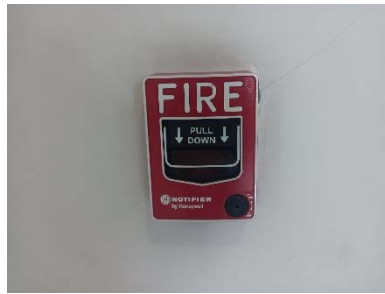
Fire Alarm Manual Station
